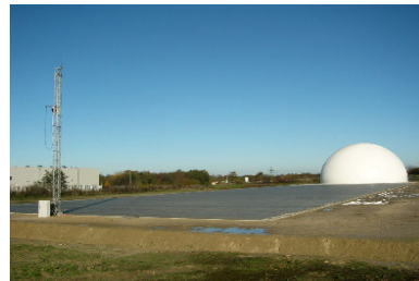
Far field tower installation
